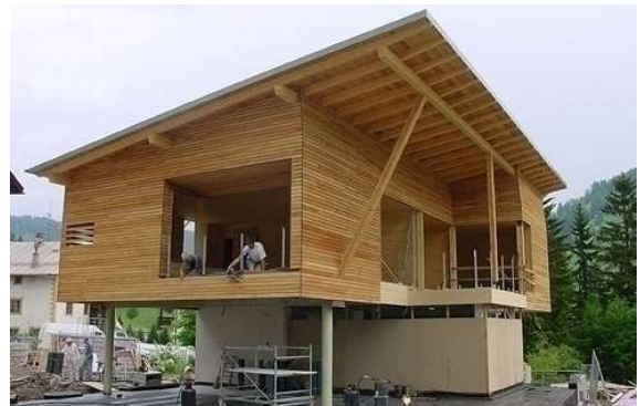
Figure 3 Thoma Holz100: connections are entirely made using dowels ("Cradle to Cradle Certified Products Registry," 2010)
