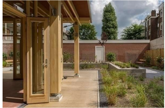
Figure 2: Accoya Wood, a biodegradable treated timber product. It comes in Radiata Pine and Alder species of wood ("Cradle to Cradle Certified Products Registry," 2010)
